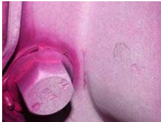
Figure 2.21. Sample #3 – End of test
