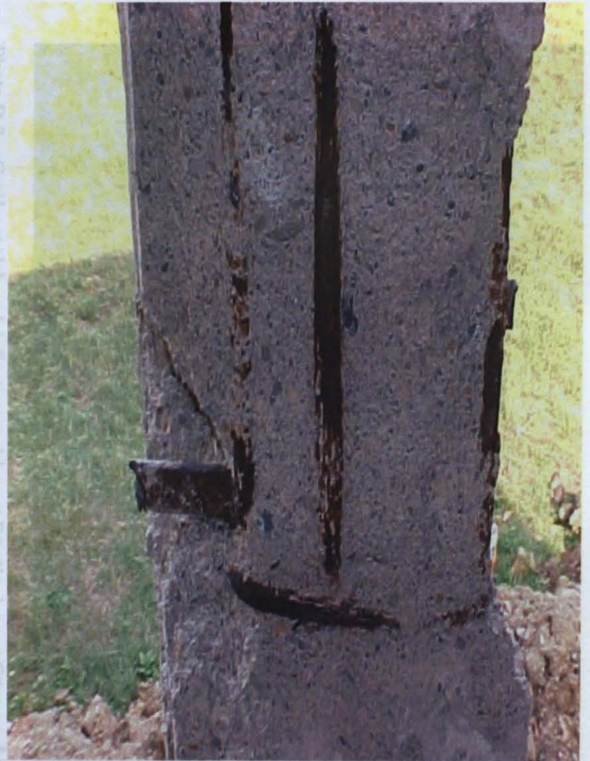
Photo D.2 – Corrosion and unconfined concrete problem at Beykoz Dereseği İ.Ö.O.
