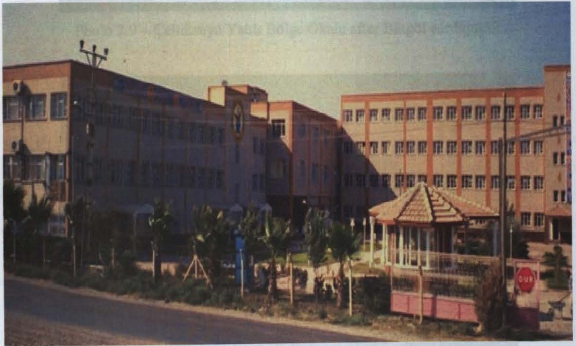
Photo 2.8 – School building west of Ceyhan with damage of grade 2 to 3
