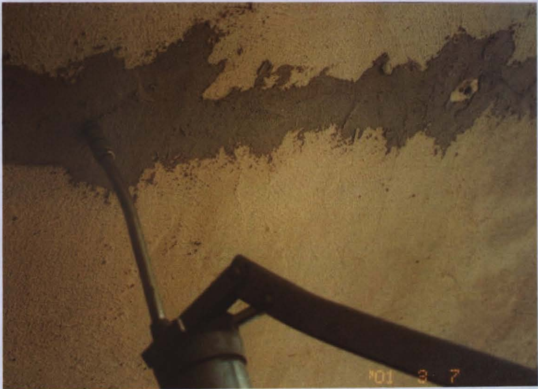
Photo D.38 – Filling the cracks with using injection of epoxy
