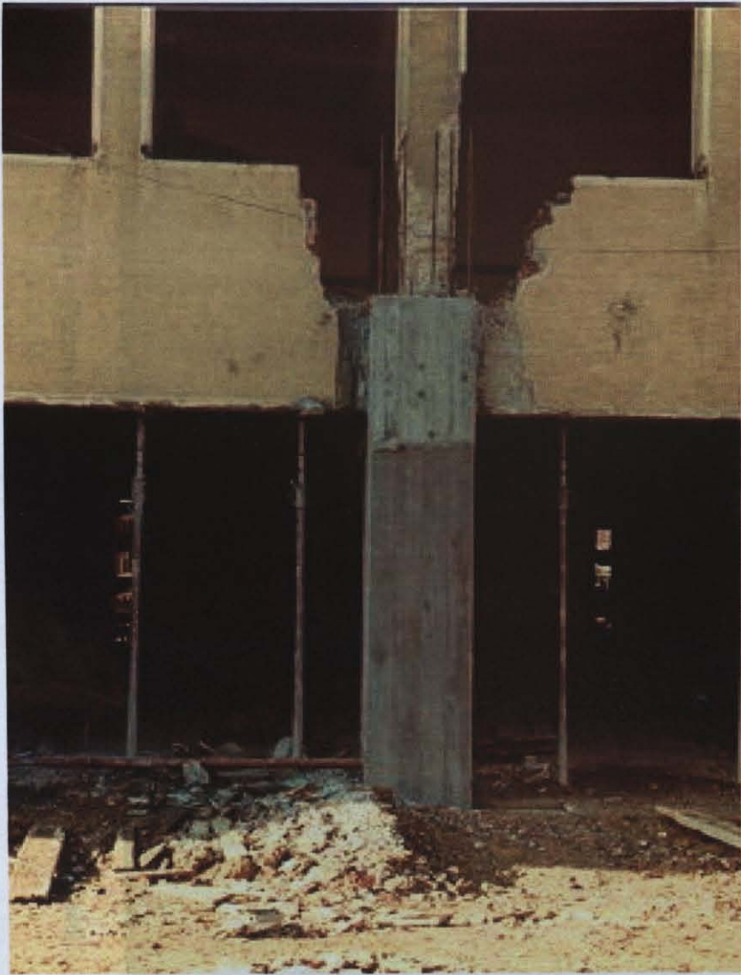
Photo D.13 – Slender column and structure design problem at Gazi Mahallesi İstiklal İ.Ö.O.
