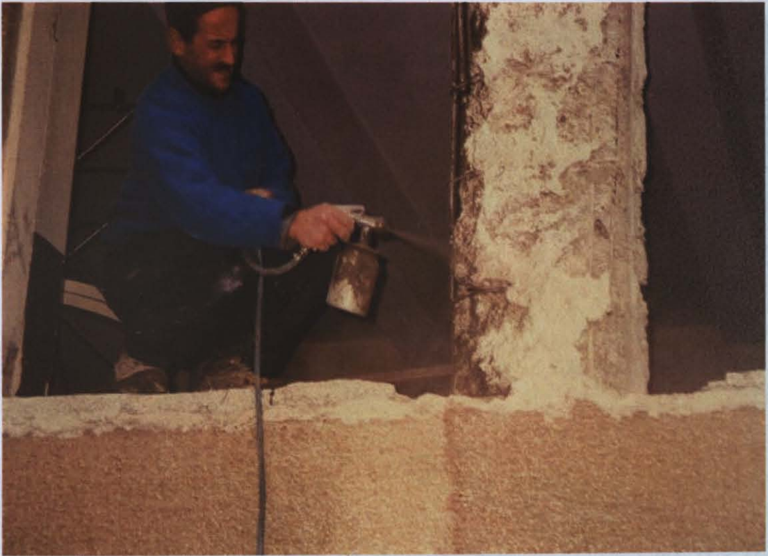
Photo D.36 – Protecting the reinforcing rebars from corrosion with protective material
