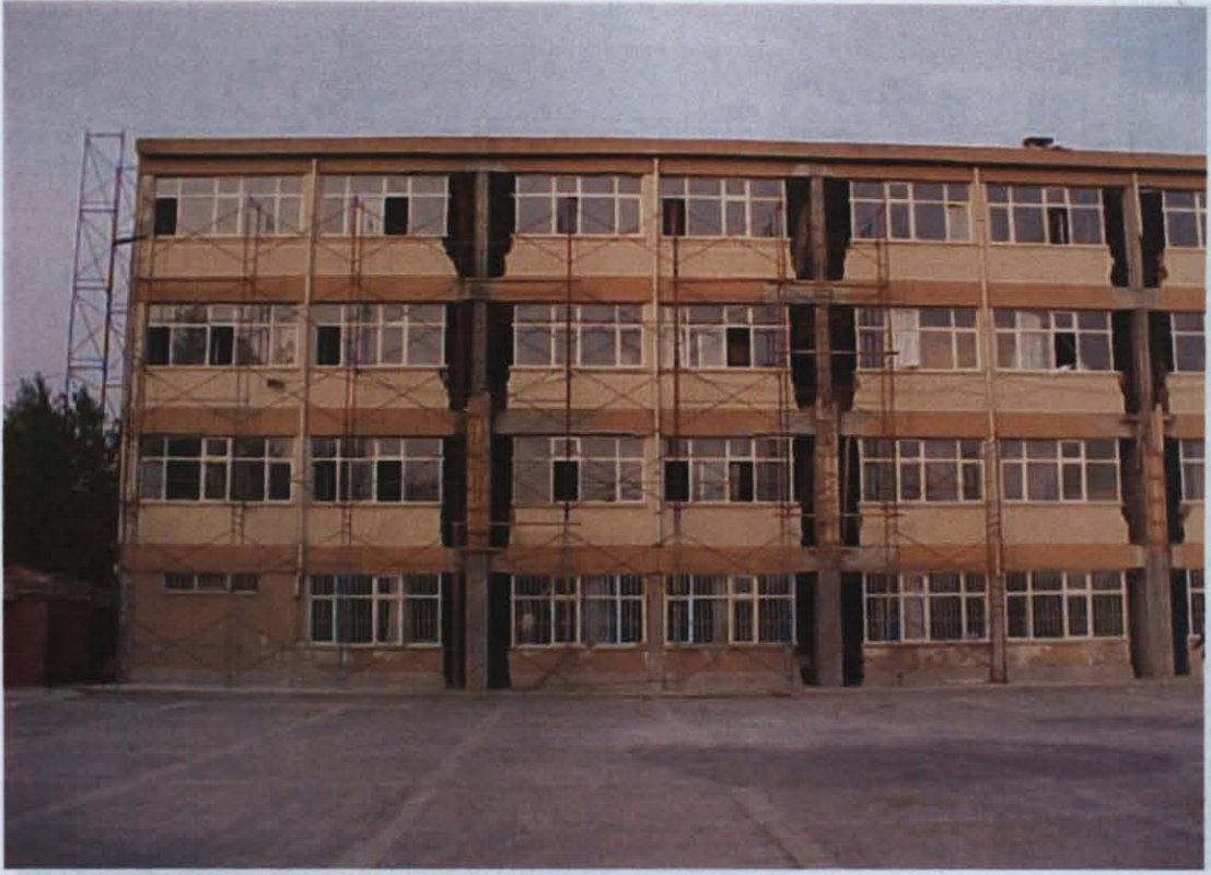
Photo D.15 – Retrofit of Kartal Anadolu Lisesi
