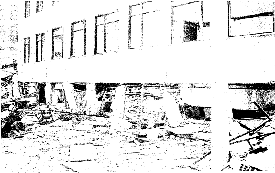
Photo 2.3 – High school building heavily damaged in Burdur earthquake
