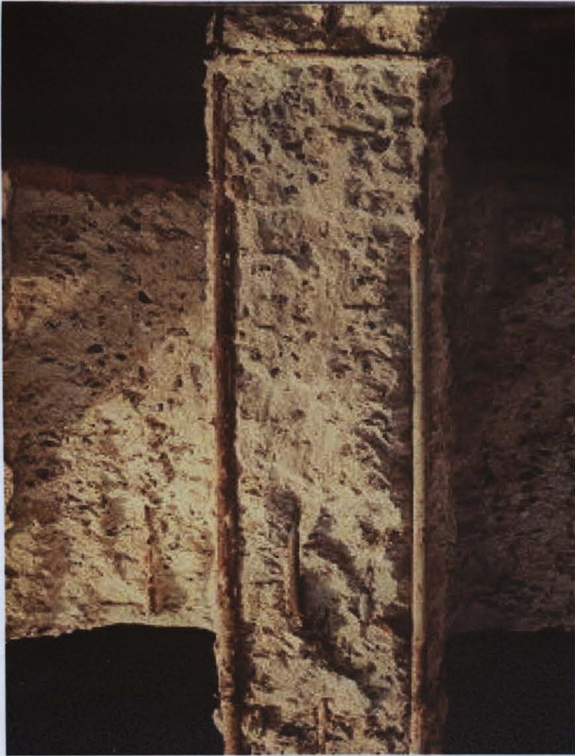
Photo D.11 and Photo D.12 – Poor quality concrete, lack of confinement and corrosion problem at Gazi Mahallesi İstiklal İ.Ö.O. Kartal Anadolu Lisesi
