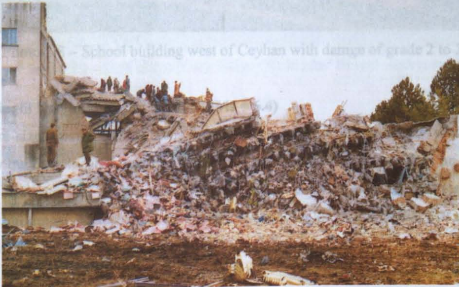
Photo 2.7 – Kız Sağlık Meslek Lisesi after Erzincan earthquake
