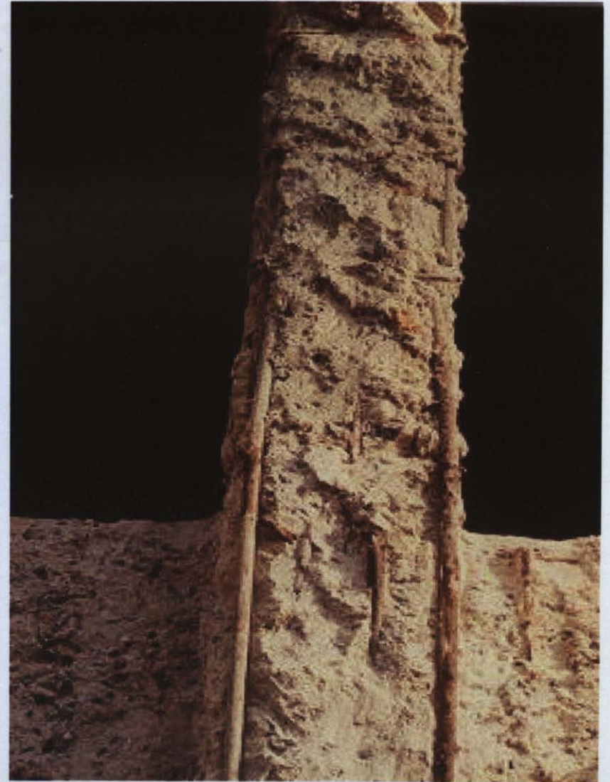
Photo D.11 and Photo D.12 – Poor quality concrete, lack of confinement and corrosion problem at Gazi Mahallesi İstiklal İ.Ö.O. Kartal Anadolu Lisesi
