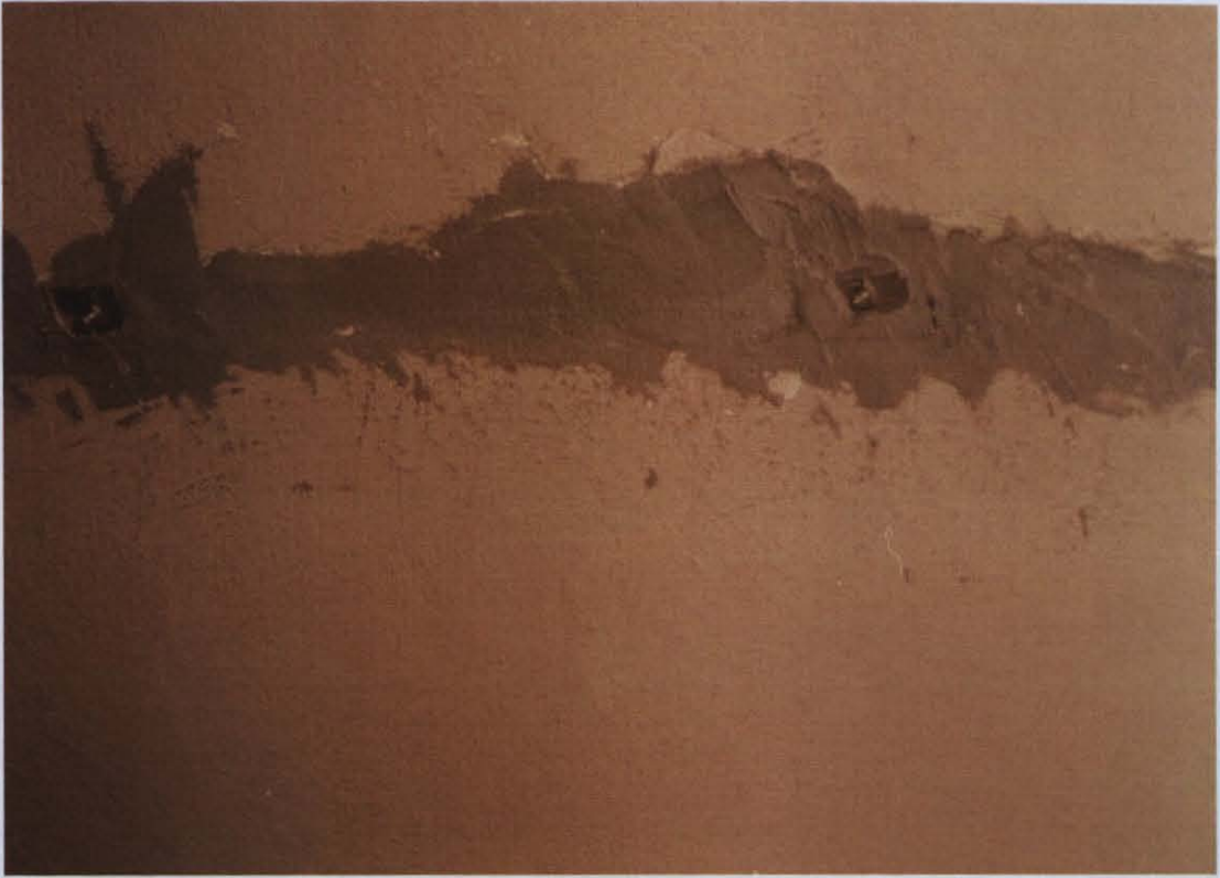
Photo D.37 – Retrofit of slab with epoxy
