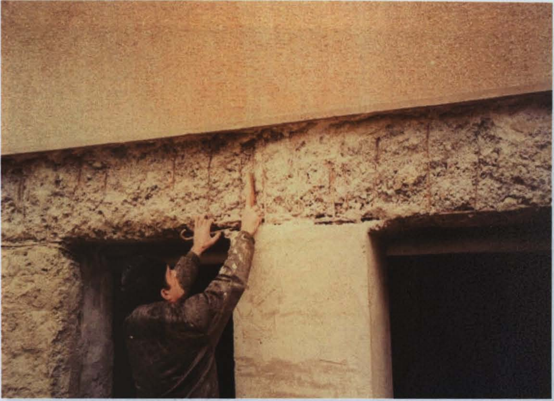
Photo D.35 – Purifying the reinforcing rebars from corrosion
