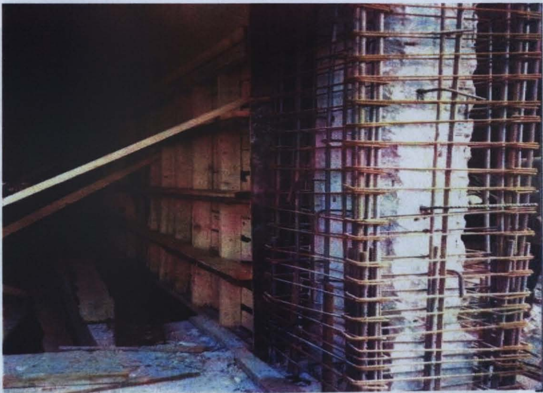
Photo D.22 – Retrofit of column at Maltepe Kaşgarlı Mahmut İ.Ö.O.
