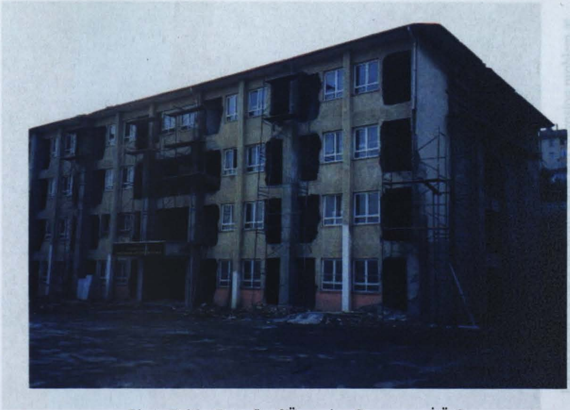
Photo D.25 – Retrofit of Ümraniye Gençosman İ.Ö.O.
