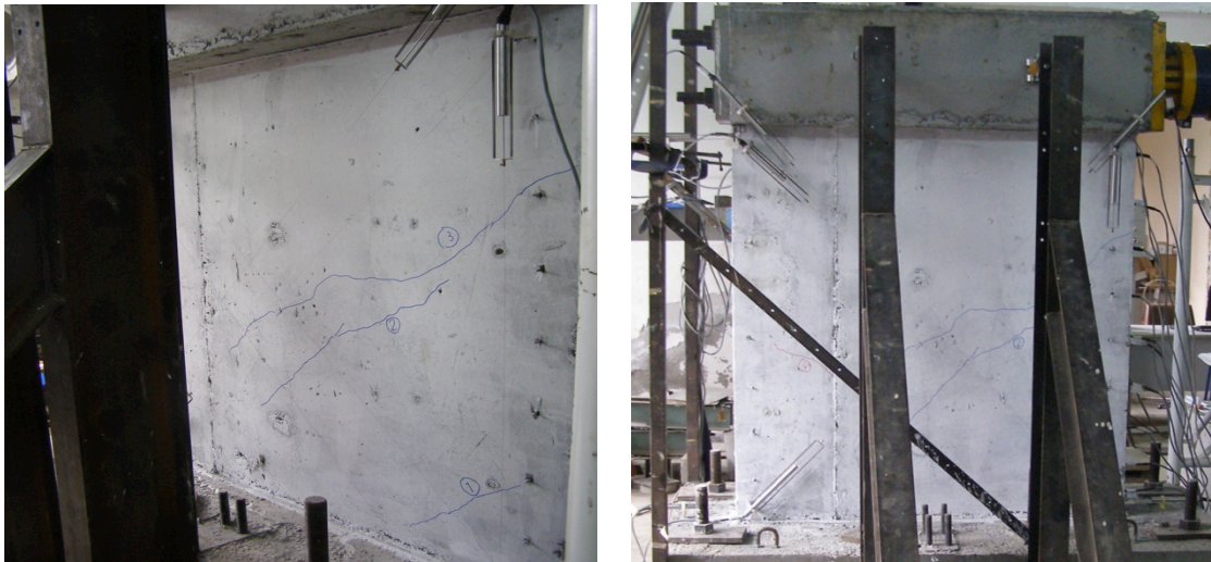
Figure 3.22. Initial Diagonal Cracks (T6-S1).
