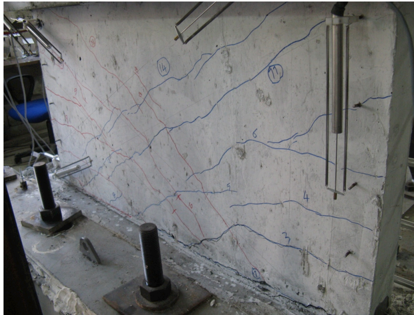
Figure 3.14. Cracking Pattern at Ultimate Load Level (T3-S1).
