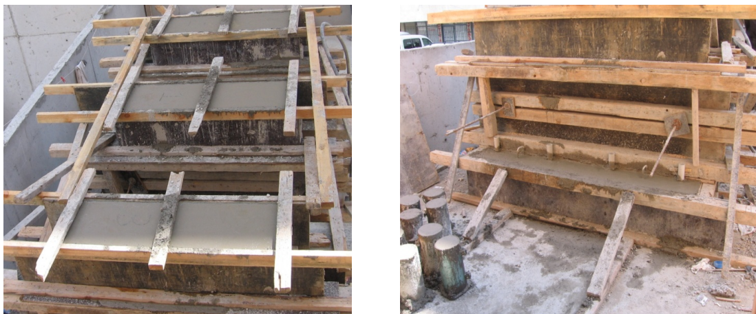
Figure 2.20. Freshly-cast concrete and cylinder specimens.
