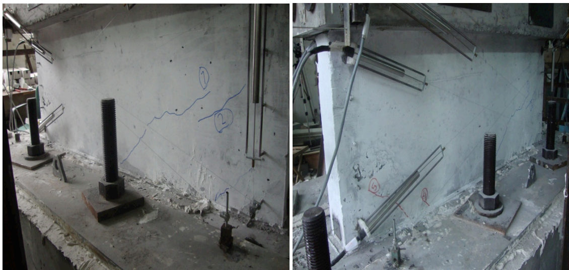
Figure 3.16. Initial Diagonal Cracks (T4-S1).
