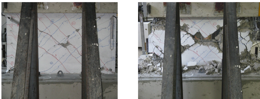
Figure 3.3. Medium and High Damage Levels (T1-S1).
