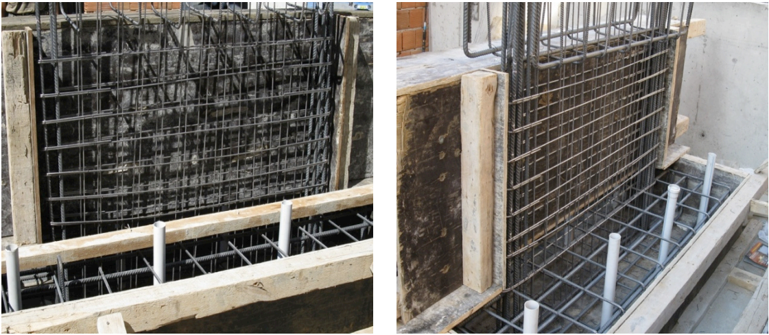
Figure 2.16. Wall and Beam Reinforcement.
