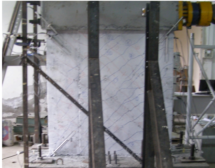
Figure 3.23. Diagonal Cracking Pattern at Ultimate Load (T6-S1).
