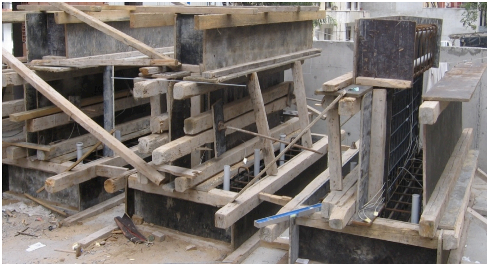
Figure 2.19. Shoring of the Formwork.
