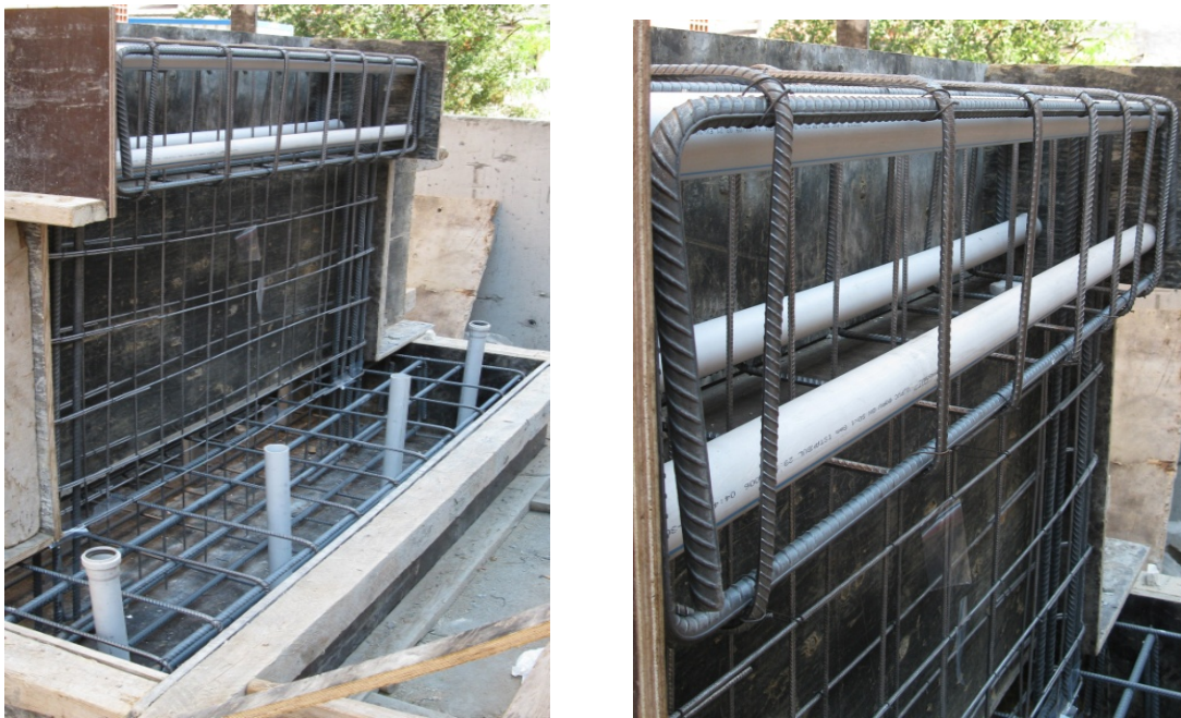
Figure 2.17. Formwork and reinforcement of Beam.
