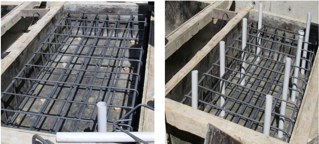
Figure 2.15. Pedestal Formwork and Reinforcement.
