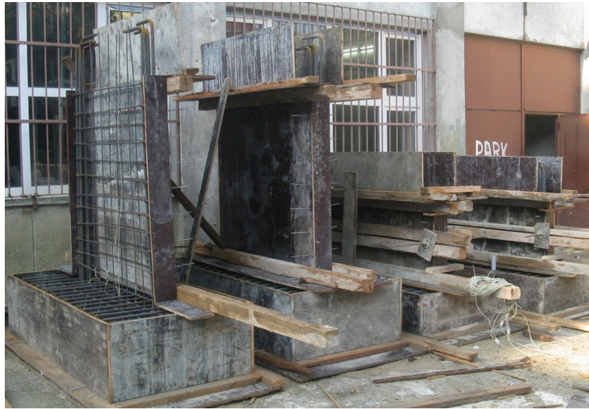
Figure 2.21. Construction of the second set of specimens.
