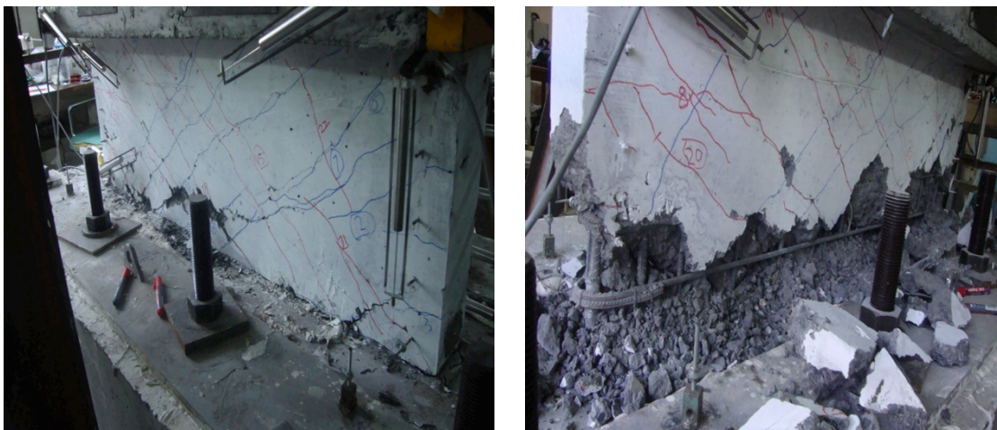
Figure 3.18. Medium and High Damage Levels (T4-S1).
