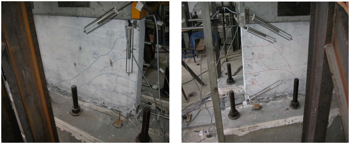
Figure 3.10. Initial Diagonal Cracks (T2-S3).
