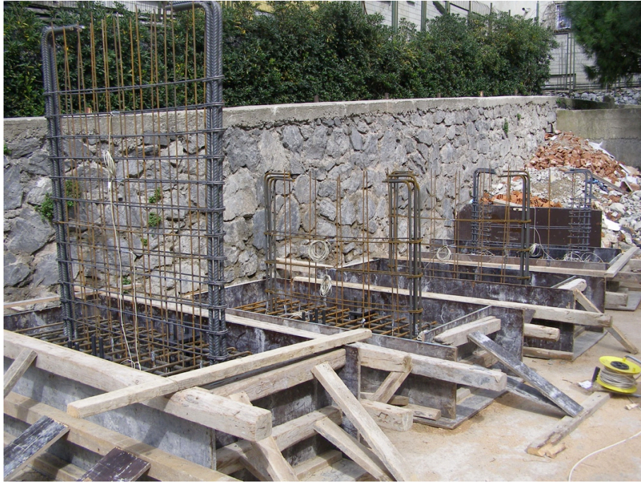
Figure 2.22. Bottom Pedestal Formwork and Wall Reinforcement.
