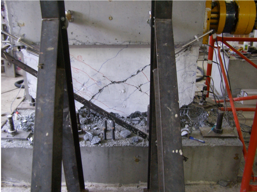
Figure 3.26. High Damage Level (T1-S2).
