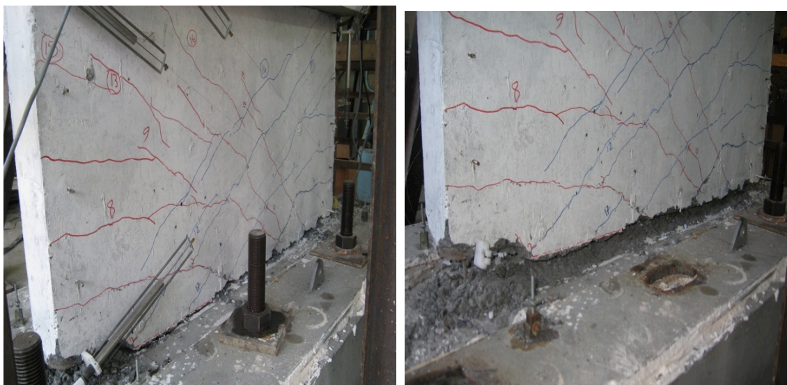
Figure 3.15. Medium and High Damage Level (T3-S1).
