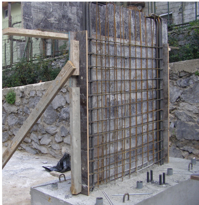
Figure 2.23. Pedestal Threaded Rods for the Axial Load Assembly.
