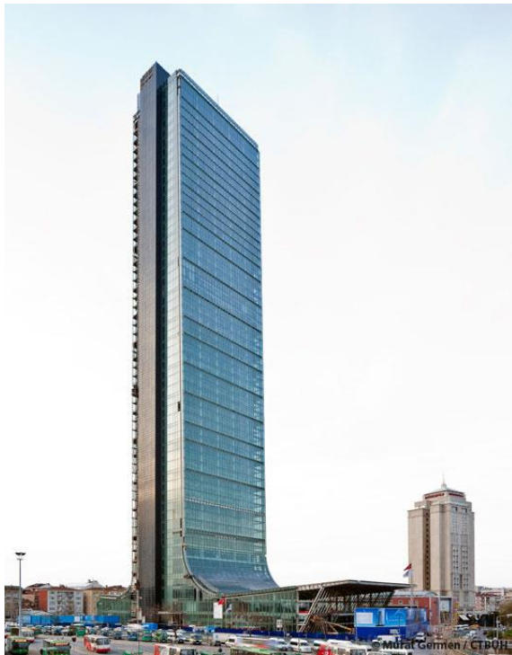
Figure 1.2. The Sapphire Building (Murat Germen, CTBUH).
