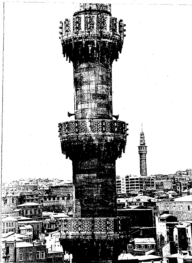
47. Yeni Cami. Detail from north-western minaret.
