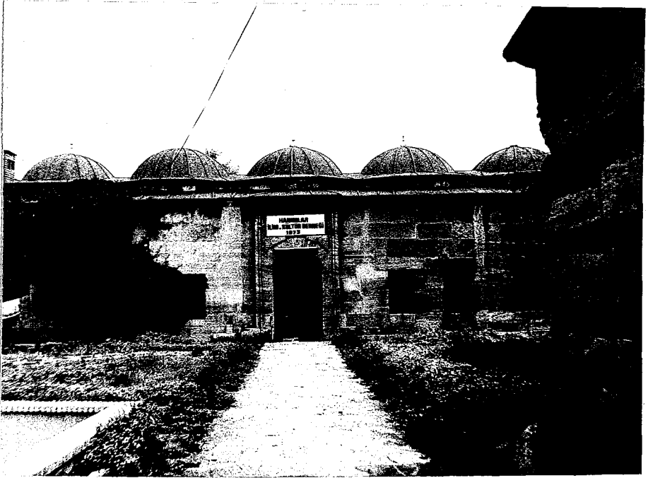
73. Bayram Paşa Complex. Outer façade of medrese.
