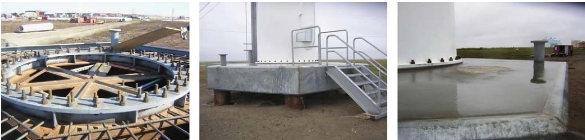
Figure 1.2. Reinforced Concrete foundation [4].
