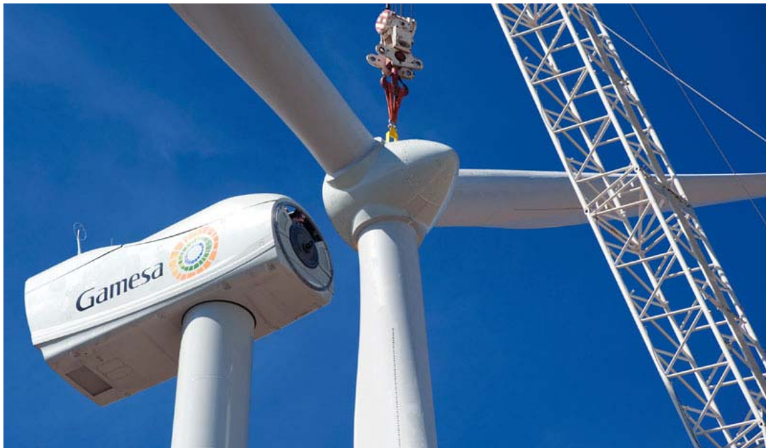
Figure 3.2. Rotor-nacelle assembly [24].
